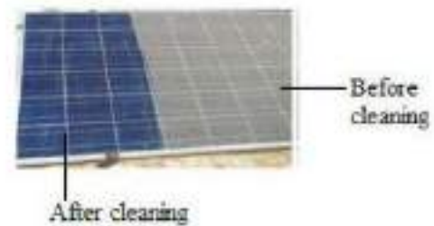
Fig.1. solar panel cleaning
